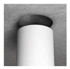
After striking the formwork, remove the formwork unit without residue from the component opening.
