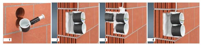
1 Make exact-fitting cable and conduit entries with the universal opening cutter Art. No. 1085-80.
